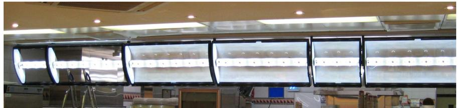
The installation used two specially manufactured brackets to fit the existing rotating menu signs. These had 3 or 6 QL4 lights, LED drivers and used the same fixings as the fluorescent brackets they were replacing. White vinyl was applied to the ends of each light fitting to increase internal reflection
